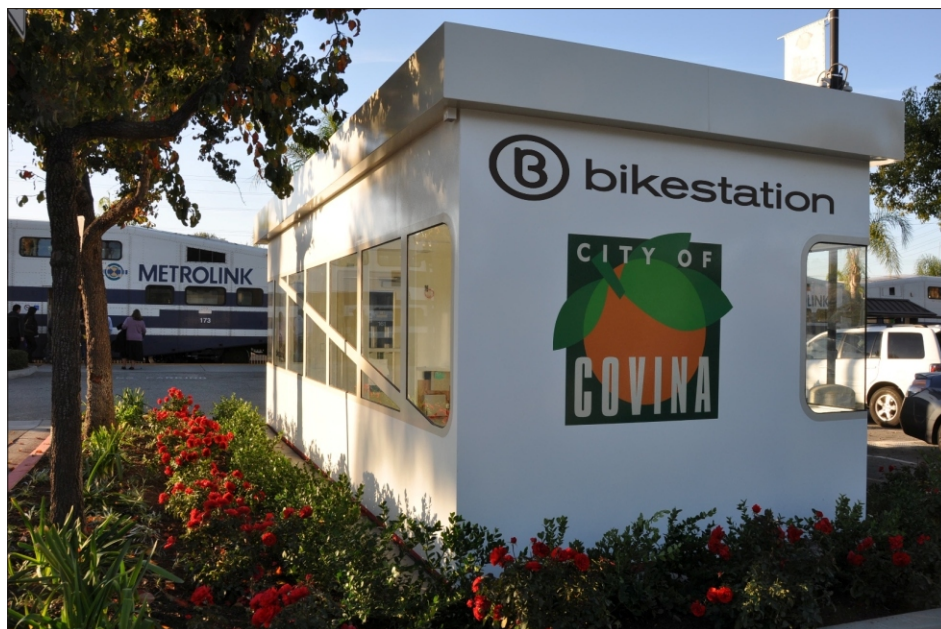
A new bikestation in Covina, CA. (Photo: Courtesy of Bikestation)
